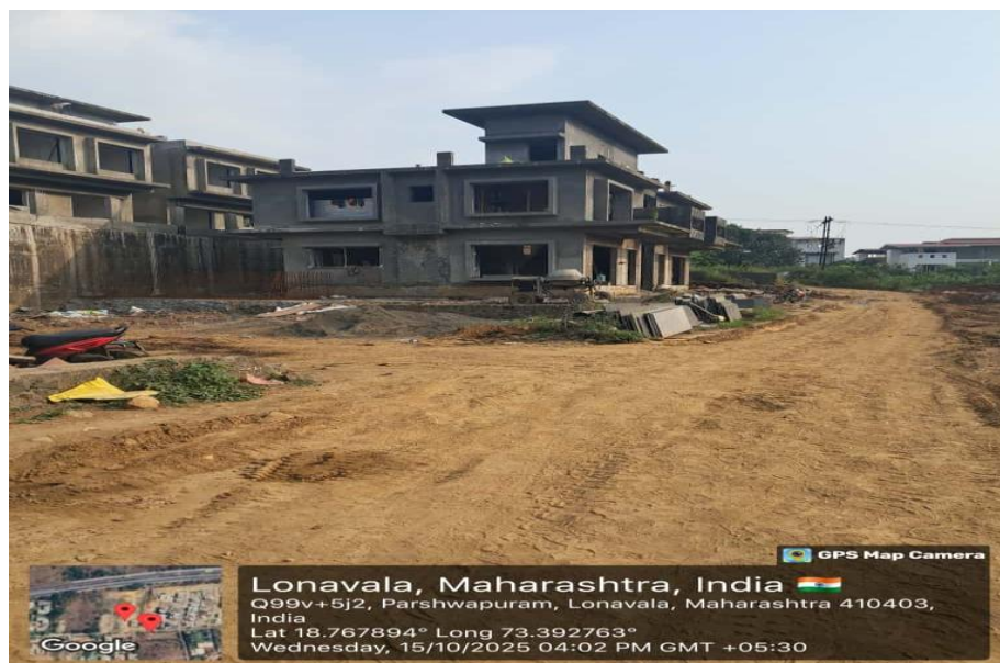
Fig. 2 Temporary road access to site
