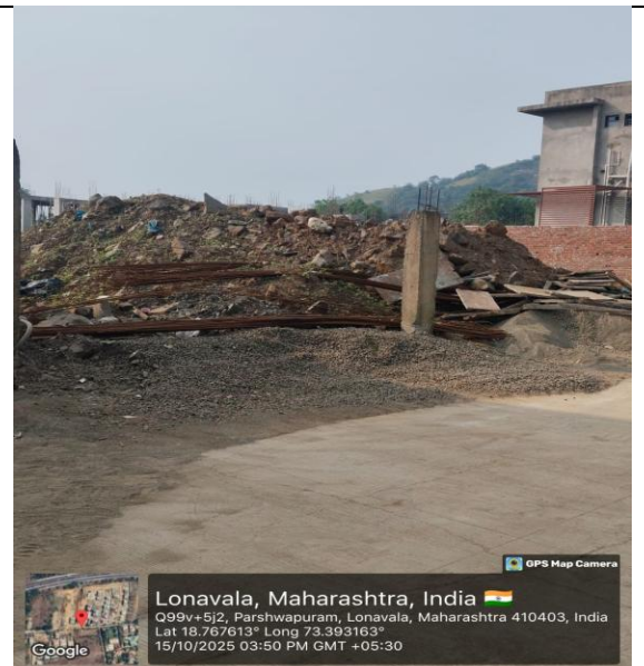
Fig. 3 Improper storage of Debris and steel
