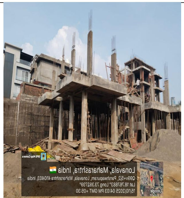
b. Material stacked closed to site
