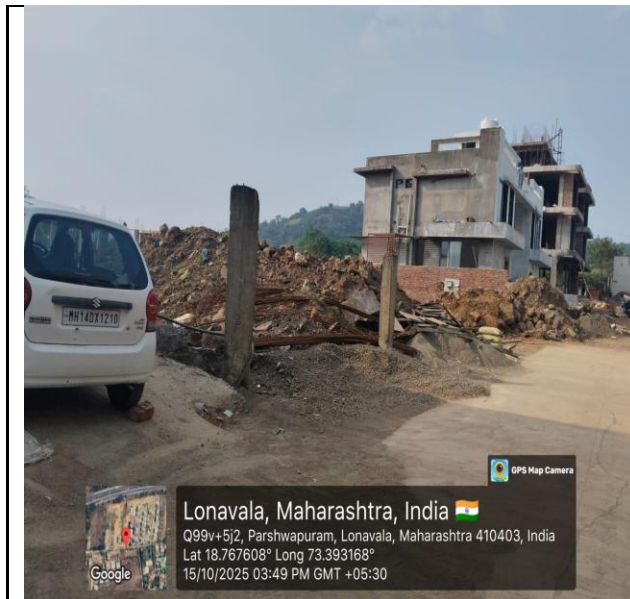
Fig. 3 Improper storage of Debris and steel
